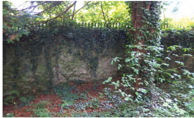
Item: Stone Boundary Wall Comments: Stone and plaster to 2.5m ht.; compromised at several locations Category: 5
