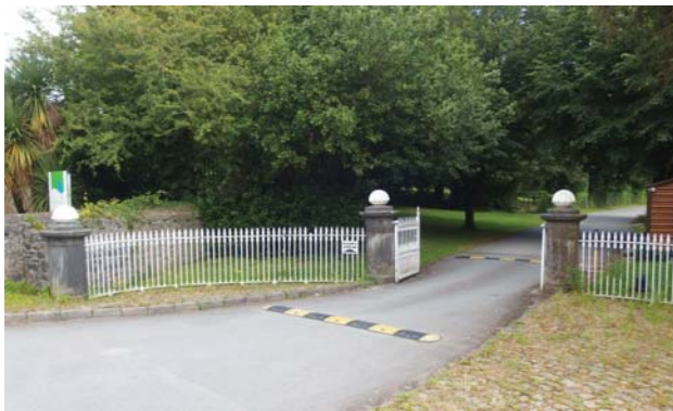
Item: Entrance Piers Comments: Scale and offset to each other Category: 4
